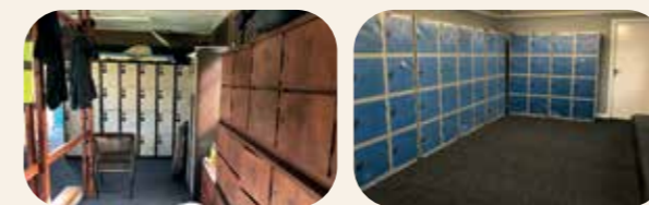
Before and after repairs
