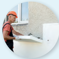
External wall insulation
