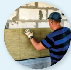
Internal wall insulation
