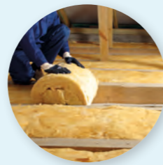
Loft insulation (including top up)
